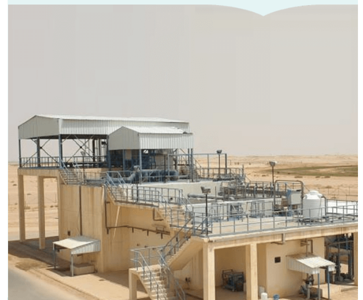
Effluent Treatment Plant (ETP) - Al Kharj
